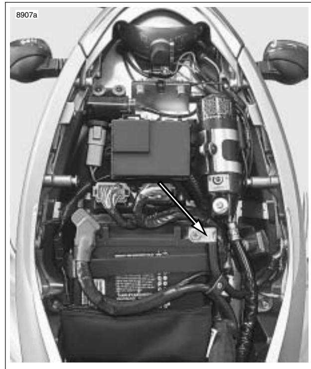
Figure 7-44. Negative Battery Cable
